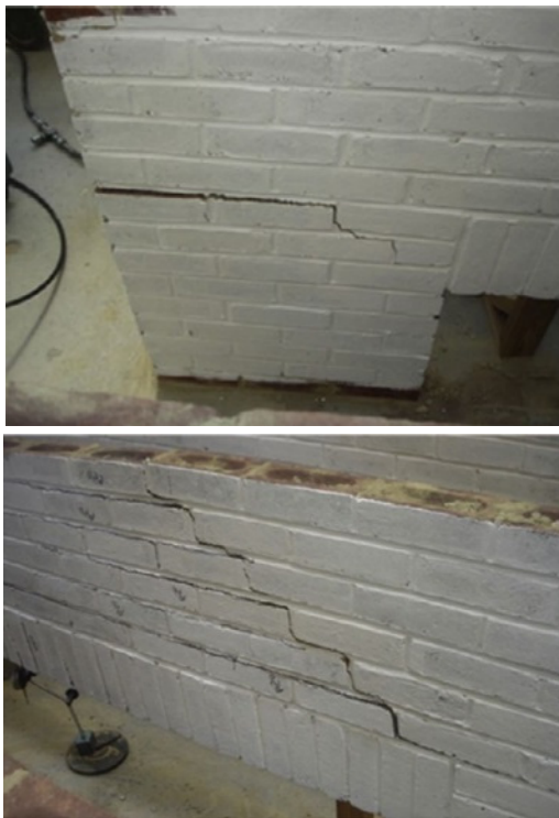
Figure 7. Typical failure mechanism of the masonry wall panel with opening (S1) as observed in the experiment.
