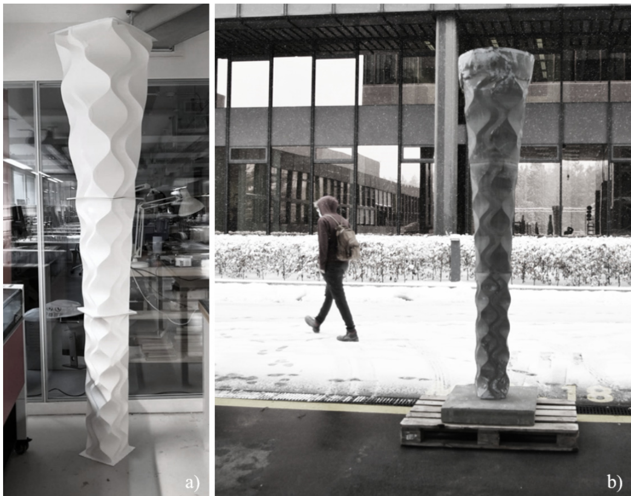
Figure 7. a), the 1 mm-thin formwork formed out of three pieces of museum board approximately 800 mm each. The resulting structure b), a tapering concrete column with a height of 2.5 -meters.
