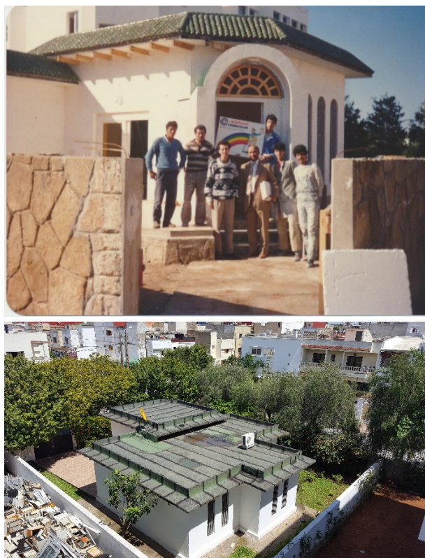
Figure 2. Experimental house made with gypsum mortar (beton Banché) (Courtsey; M. Sonebi, 1989 and 2018).
