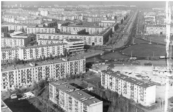
Figure 1. Example of Ukrainian building stock of prefabricated structures produced in the 1960-1970s. Darnytska Square, Kyiv, 1966s. Source: http://starkiev.com/
