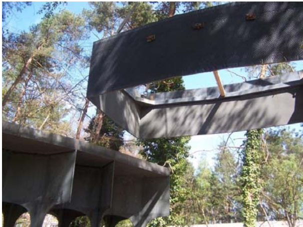
Figure 4. FIFA World Cup Pavilion, City of Kaiserslautern, Germany – mounting the attic.
