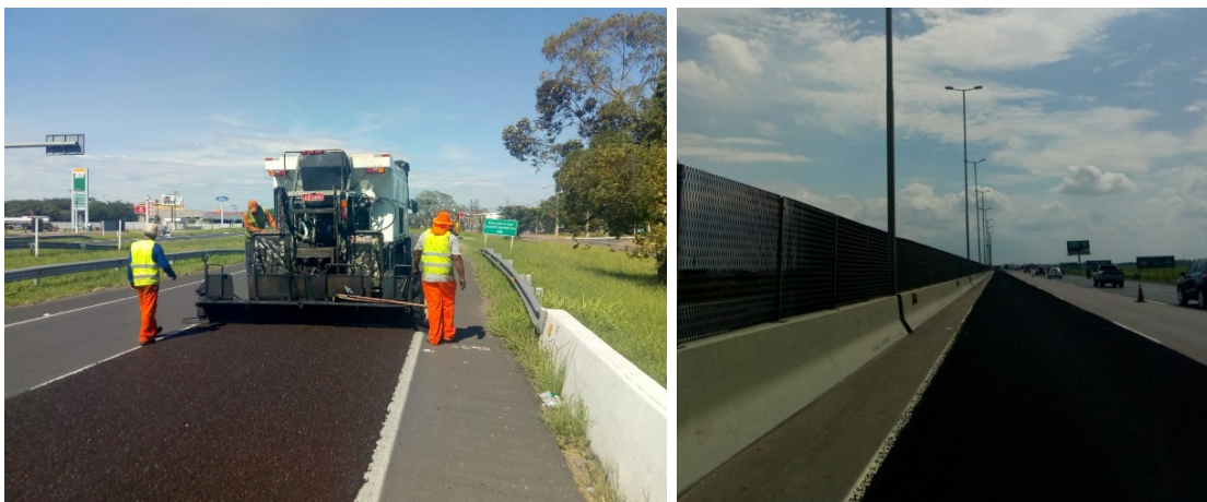
Figure 5. Microsurfacing on high traffic highway, during and after construction.
