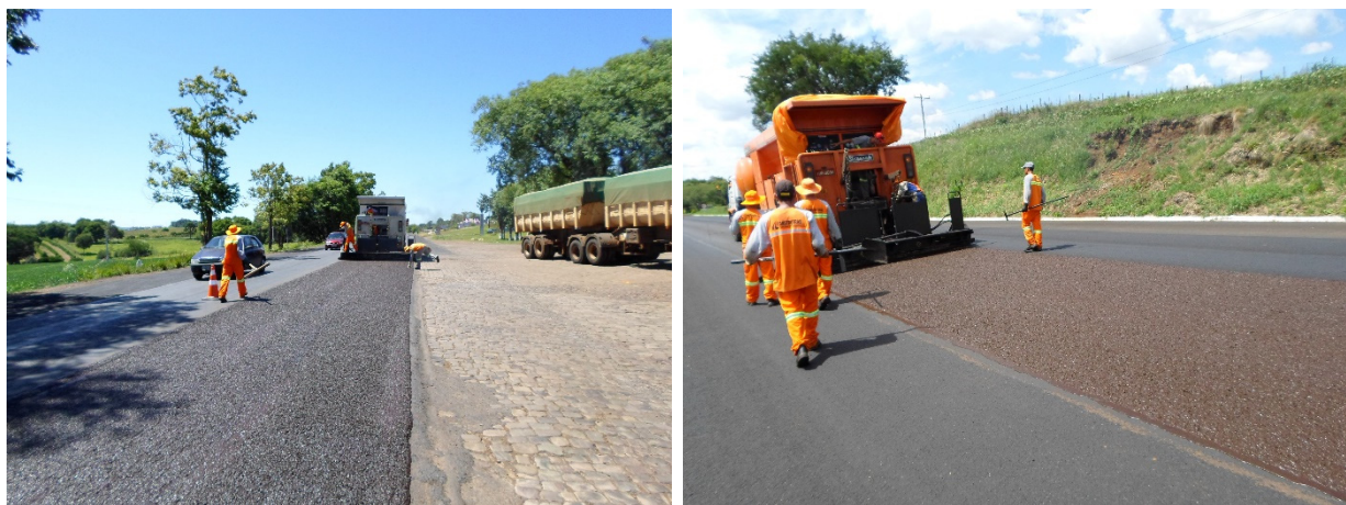
Figure 3. Example of an application of microsurfacing in Brazil.
