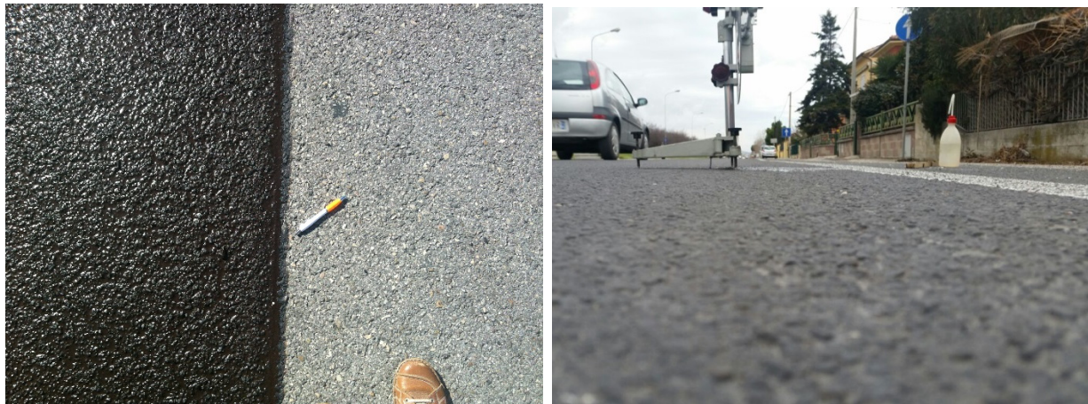
Figure 2. Example of an application of BSS in fresh state and after setting in Italy.
