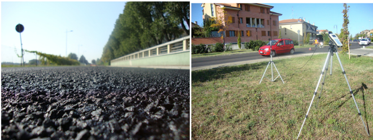
Figure 6. Multifunctional microsurfacing in Ozzano Emilia (Bologna, Italy).
