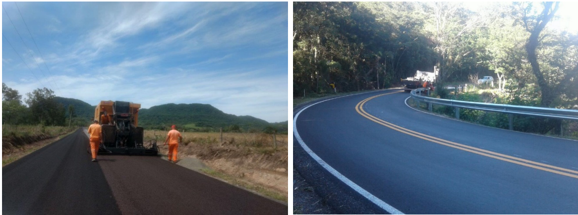
Figure 4. Microsurfacing on VRS-804 road during and after construction.
